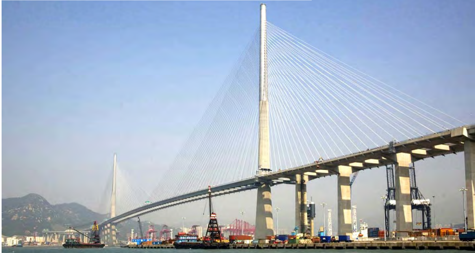
Stonecutters Bridge, Hong Kong
