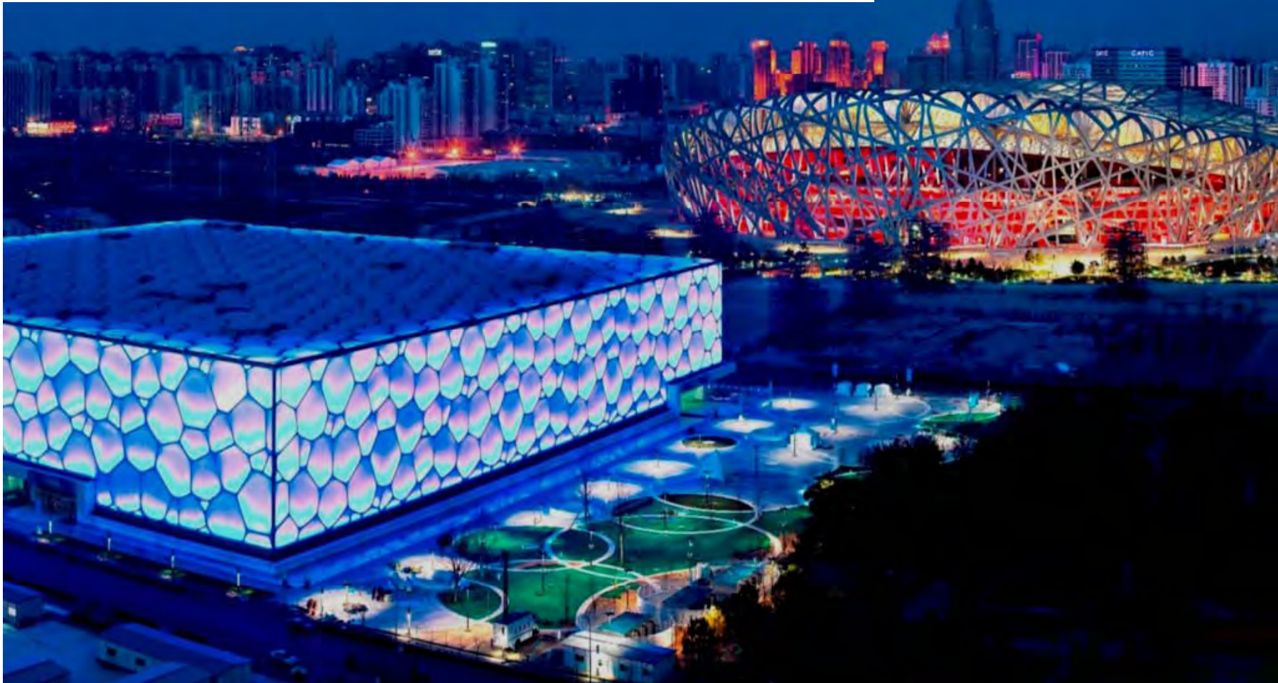
Beijing National Stadium & National Aquatics Centre
