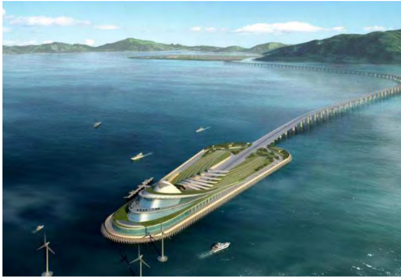
Hong Kong-Zhuhai-Macau Bridge, China
